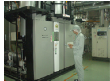
High-efficiency, high-pressure once-through boiler
